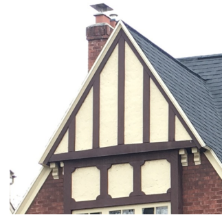
Corbels under jetty
